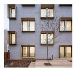
Deeply recessed windows with projecting linings to CSB first floor laboratories
