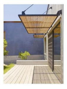
Vertical timber fins supported by anodised aluminium frames will provide solar shading to deal with the low angle sun
