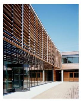
Solar shading to the entrance building will be a vertical array of horizontal timber aerofoil section fins
